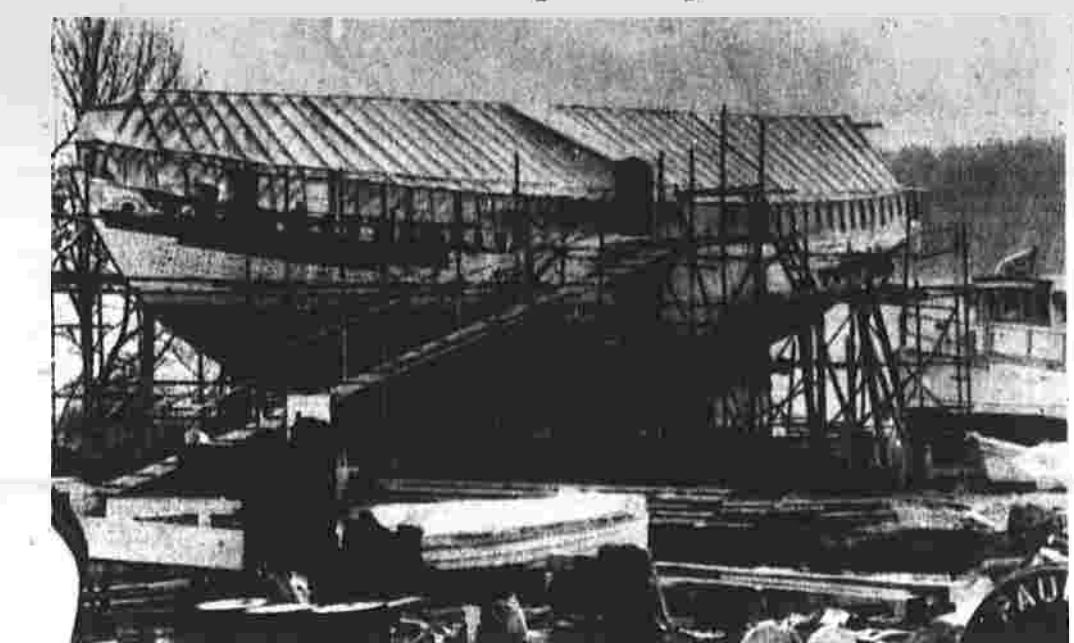
The famed schooner Bowdoin sits on the ways of the Percy and Small Yards in Bath, Maine, undergoing extensive restoration work. The work is being funded by a matching grant from the National Trust for
